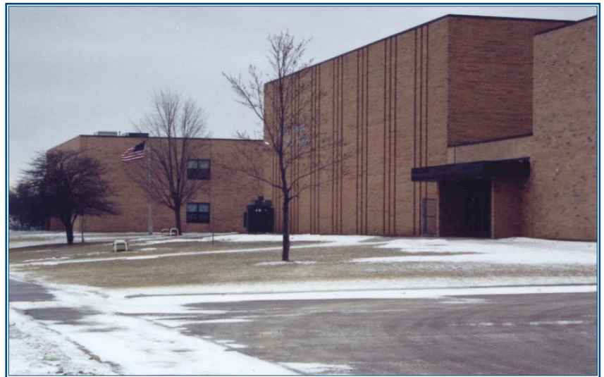
Tomah High School is one of nine schools in the district where half a million square feet of carpet is maintained with the HOST ® Dry Extraction Carpet Cleaning System.
